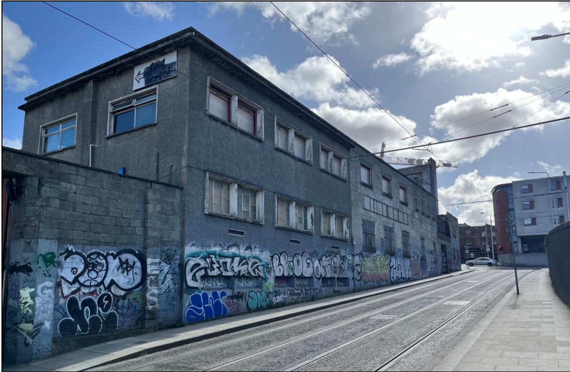
Plate 15: Warehouse building (B3)
