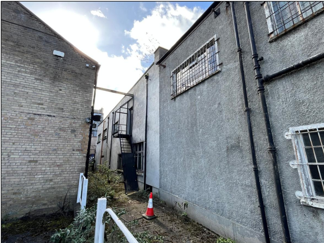
Plate 16: Warehouse building (B3)
