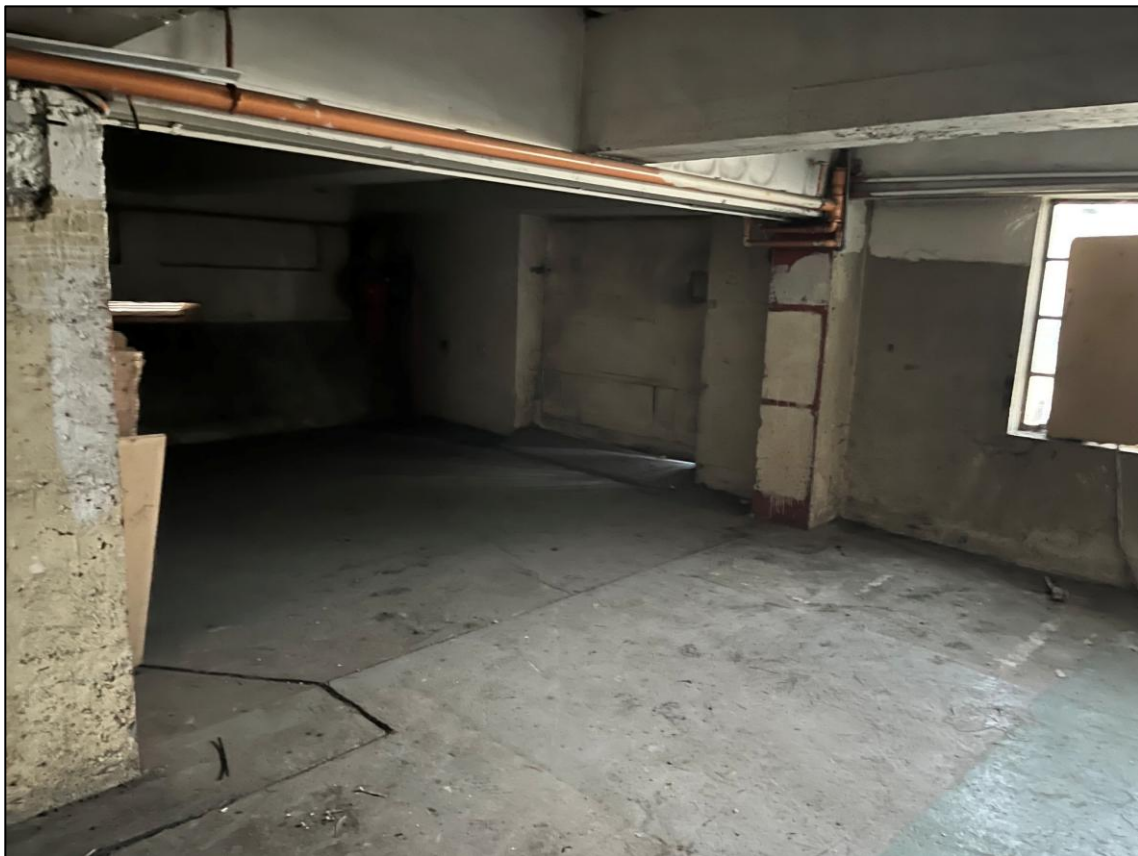
Plate 18: Warehouse building (B3) internals
