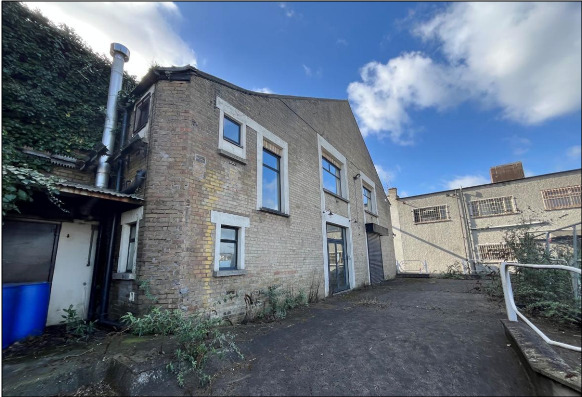
Plate 5: Office building (B2)
