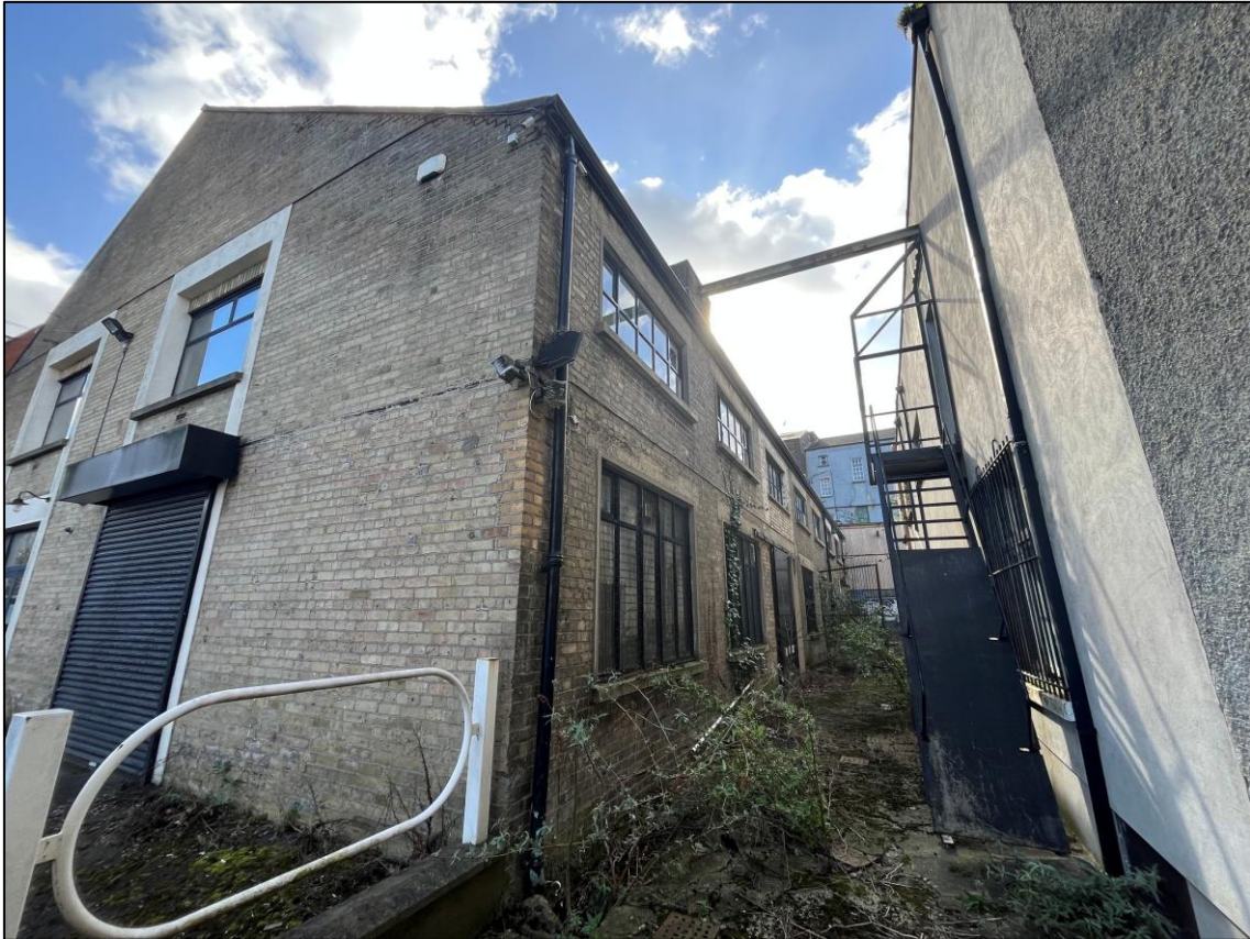
Plate 7: Office building (B2)
