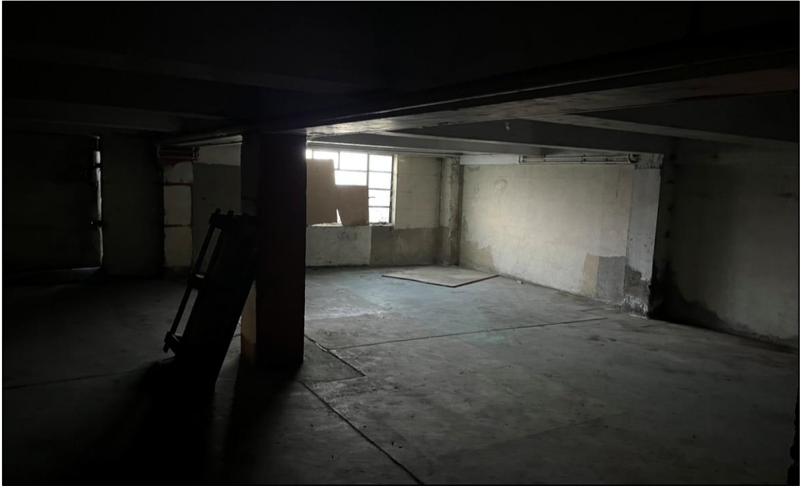
Plate 17: Warehouse building (B3) internals
