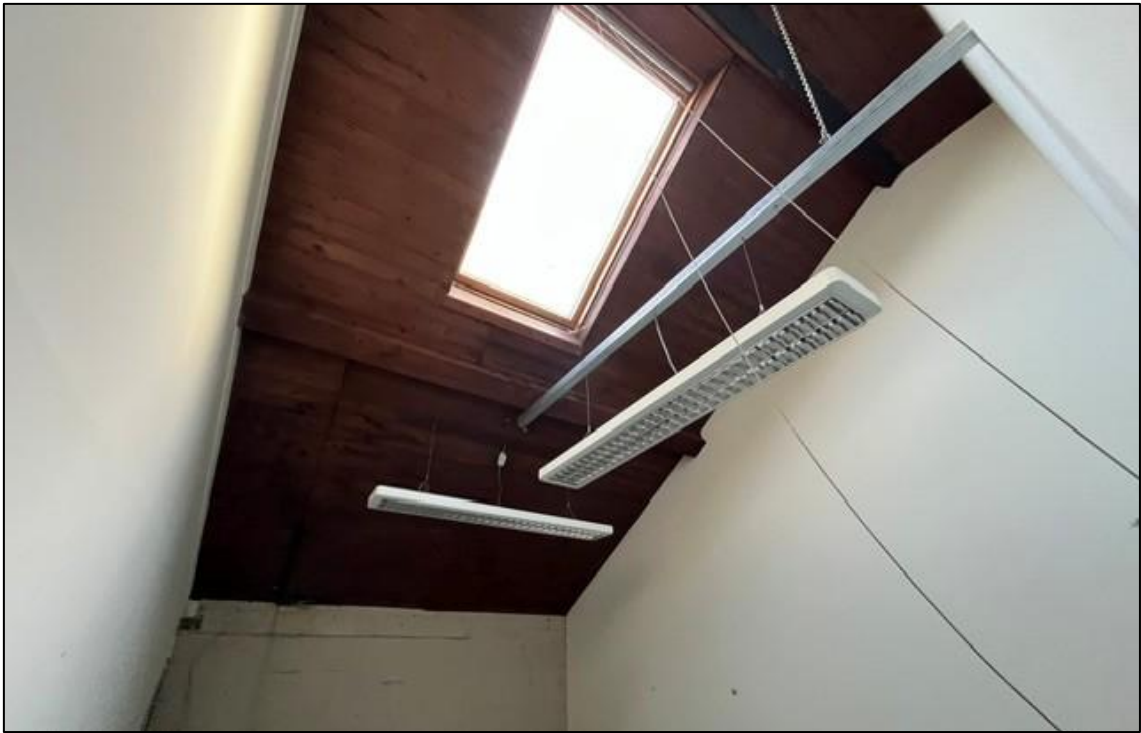
Plate 11: Office building (B2) internals
