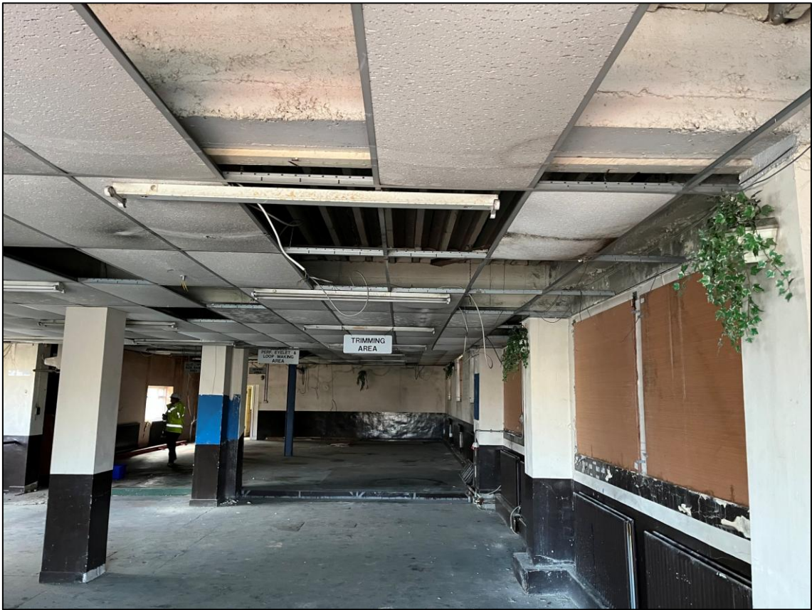
Plate 12: Office building (B2) internals
