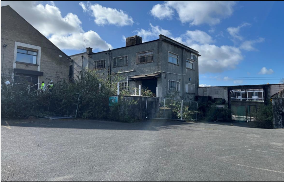
Plate 19: Example of hard standing and vegetation found on site.
