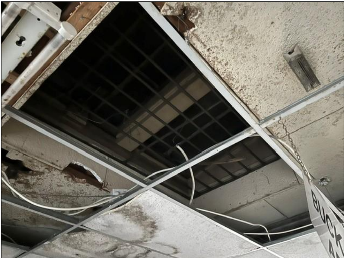
Plate 10: Office building (B2) internals
