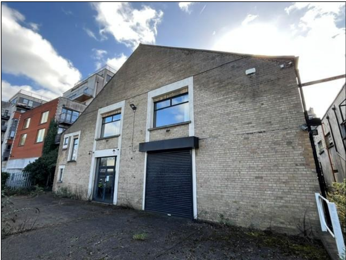
Plate 6: Office building (B2)
