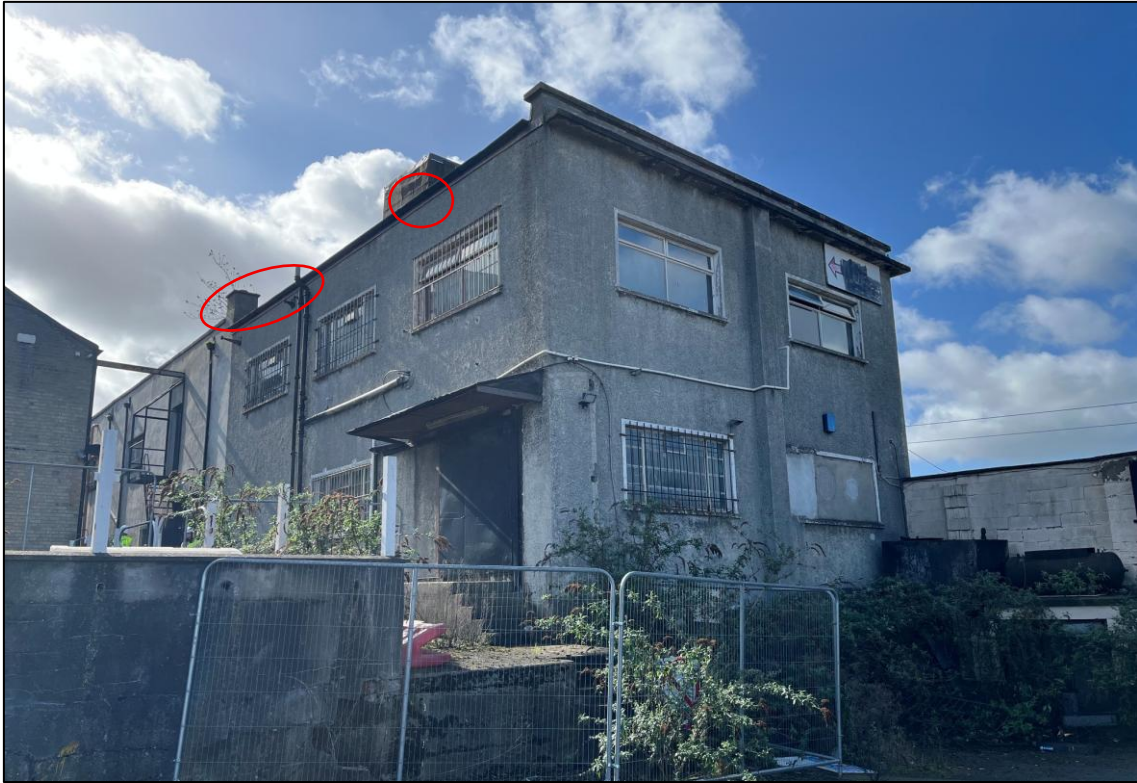
Plate 13: Warehouse building (B3)
