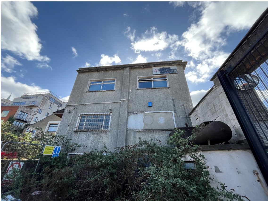
Plate 14: Warehouse building (B3)
