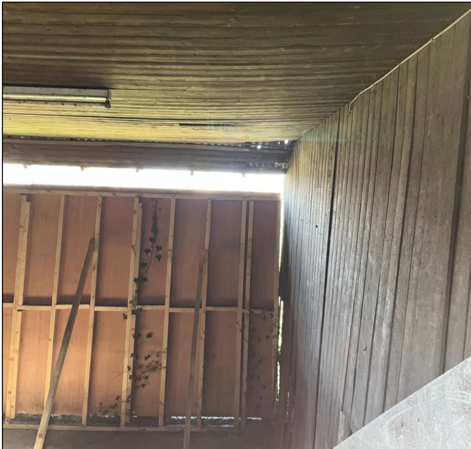
Plate 4: Shed building (B1) internals
