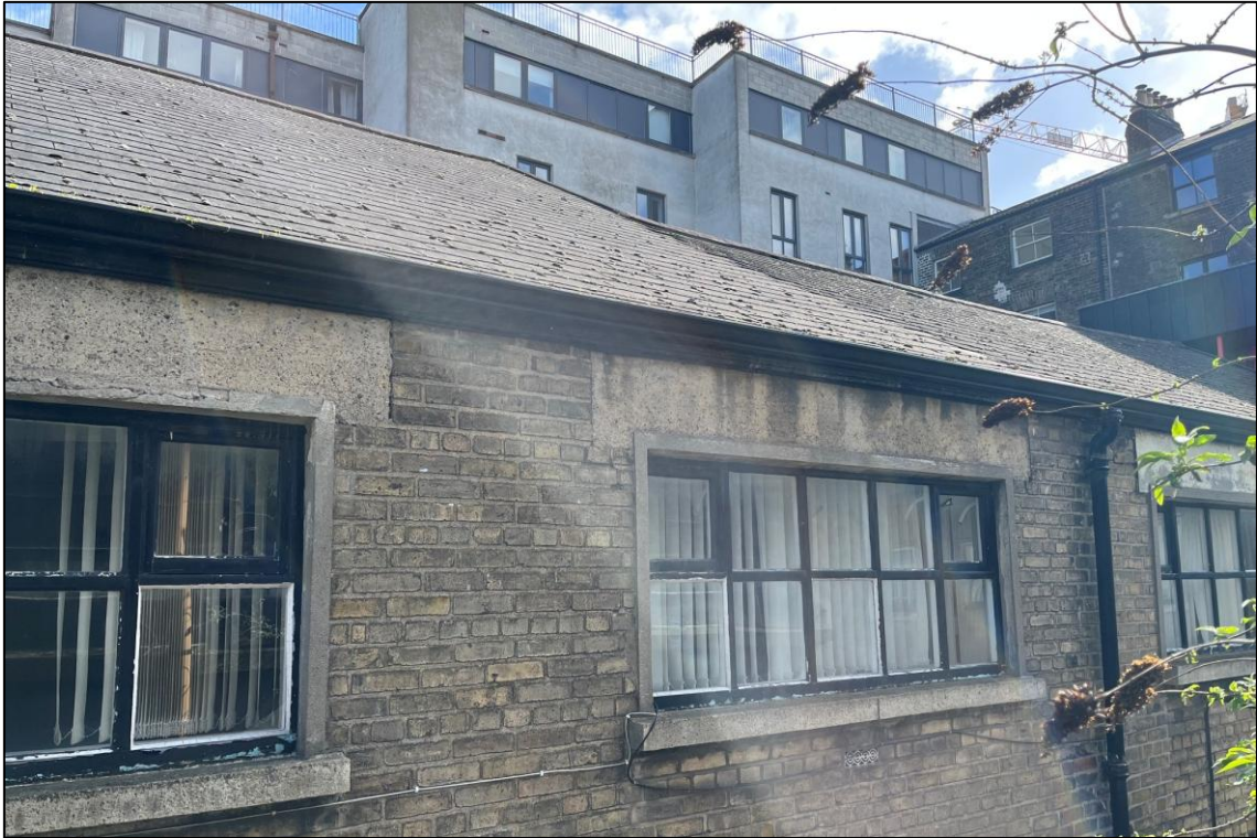
Plate 9: Office building (B2) - Tight fitting slate roof tile present.
